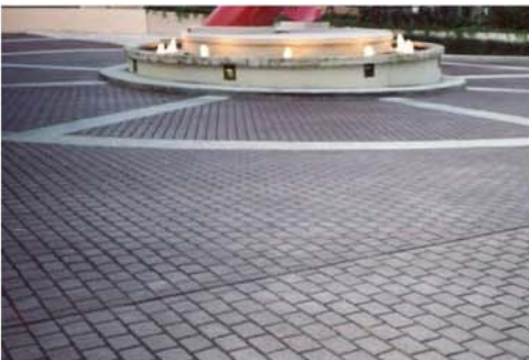
New Brick Running Bond M-151
